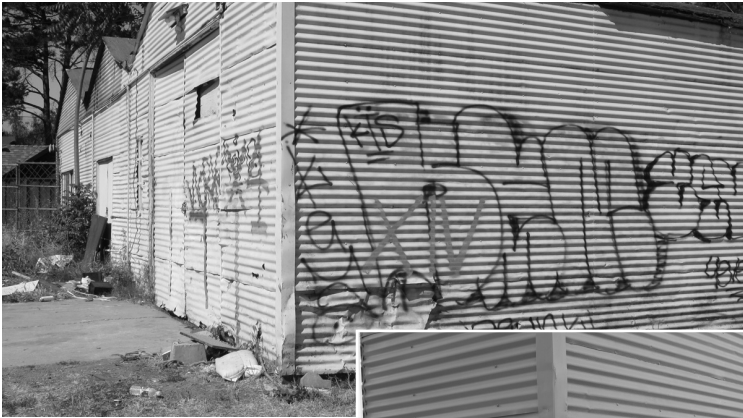
Bob uses five different kinds of removal spray, and has to date removed at least 12,500 tags! A before shot of the tagged building at 505 Barron Ave. which is scheduled to become "Keep it Secret."
