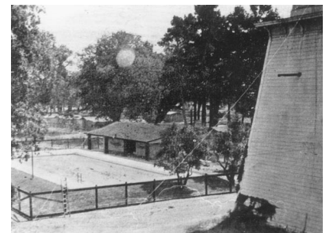
Water Tower with Pool in Background.
