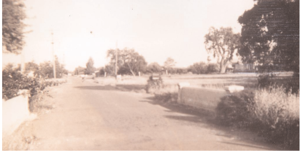
Laguna Avenue, 1946—looking towards Los Robles from the Matadero Creek Bridge.
